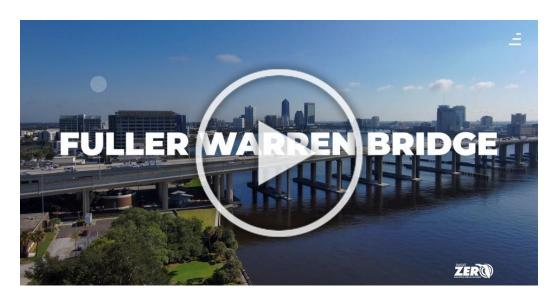
Spanning the St. Johns River at 4,654 feet long and 12 feet wide, the Fuller Warren SUP includes two 6-foot lanes for east/west traffic and features two rest/observation
